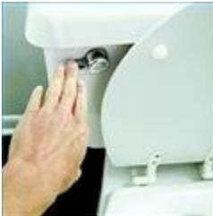
Open the shut off valve and allow the tank to fill and then test with a series of flushes to inspect for leaks or water backups.
