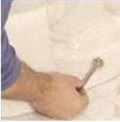
Secure the bolts by hand tightening them to the floor use caution when you do this as over tightening can cause porcelain to crack. Use caulk or plumbers putty to apply a seal around the base of the toilet and the respective bolts.
