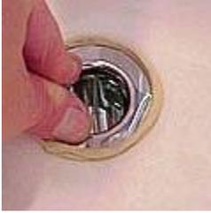
Prior to installing the new drain, take a bit of plumbers putty and roll it between your palms so that it forms a long "snake" of putty of sufficient length to wrap around the drain. Press the putty onto the underside of the new drain flange and insert the drain into the sink. The plumbers putty will squeeze out from around the drain flange. You can remove the excess later.
