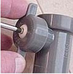
Under the sink, insert the pop up drain control rod into the back of the drain tailpiece as depicted by the picture above. Then tighten on the securing nut as depicted by this picture.
