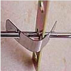
Finally attach the pop up lever to the control rod as depicted. Clean off all plumber's putty and test!
