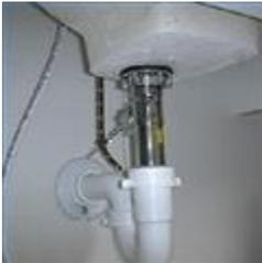
Start by clearing out under the sink so that you have ample room to work. Under the sink, you will see that the drain is actually connected into the trap (a U shaped portion of pipe) by a compression cap. Loosen the cap so that the drain will slide up and out.
