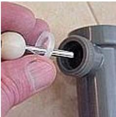
Insert the lever for the pop up drain through the back of the faucet and insert the pop up into the drain.
