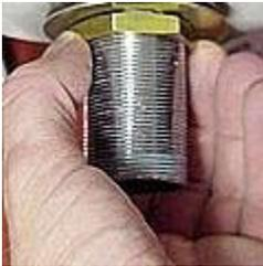
Next, secure the drain to the sink from the underside by installing the large gasket and nut. Hand tighten as far as possible, then use your wrench or pliers to snug everything up. Be careful not to over tighten as you could crack the sink.
